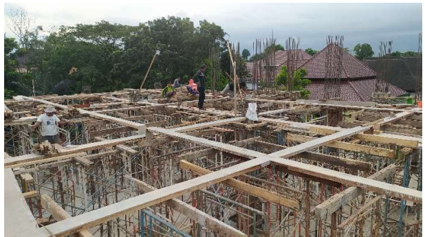
Bodeman Balok Lantai Rooftop
