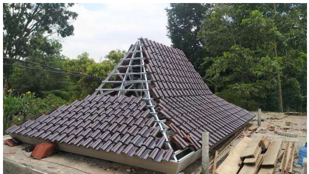
Pemasangan Genting Glazur atap drop off area
